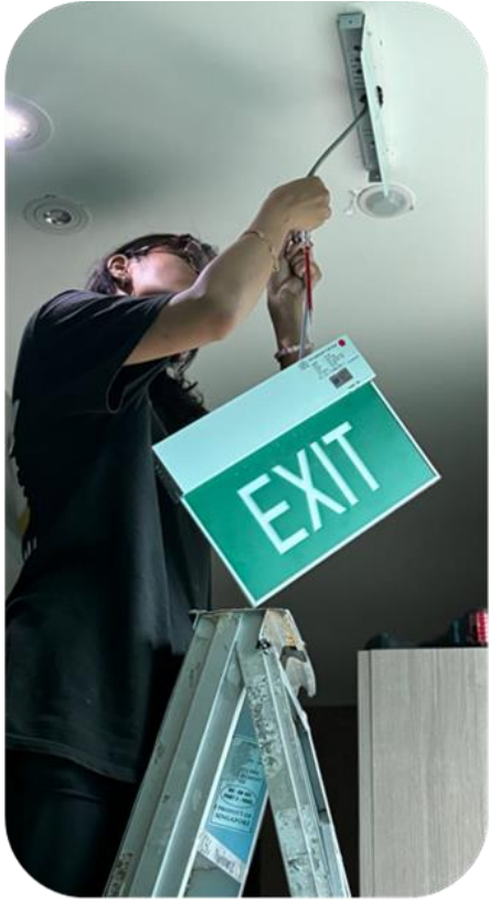
Installing Emergency Exit Light @ Civil Service Club
