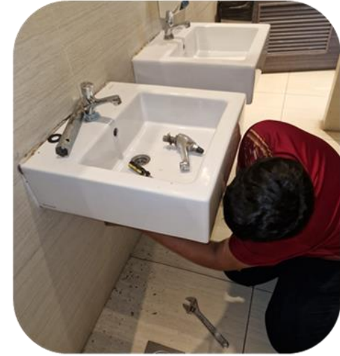
Replacing Water Faucet @ HomeTeam NS
